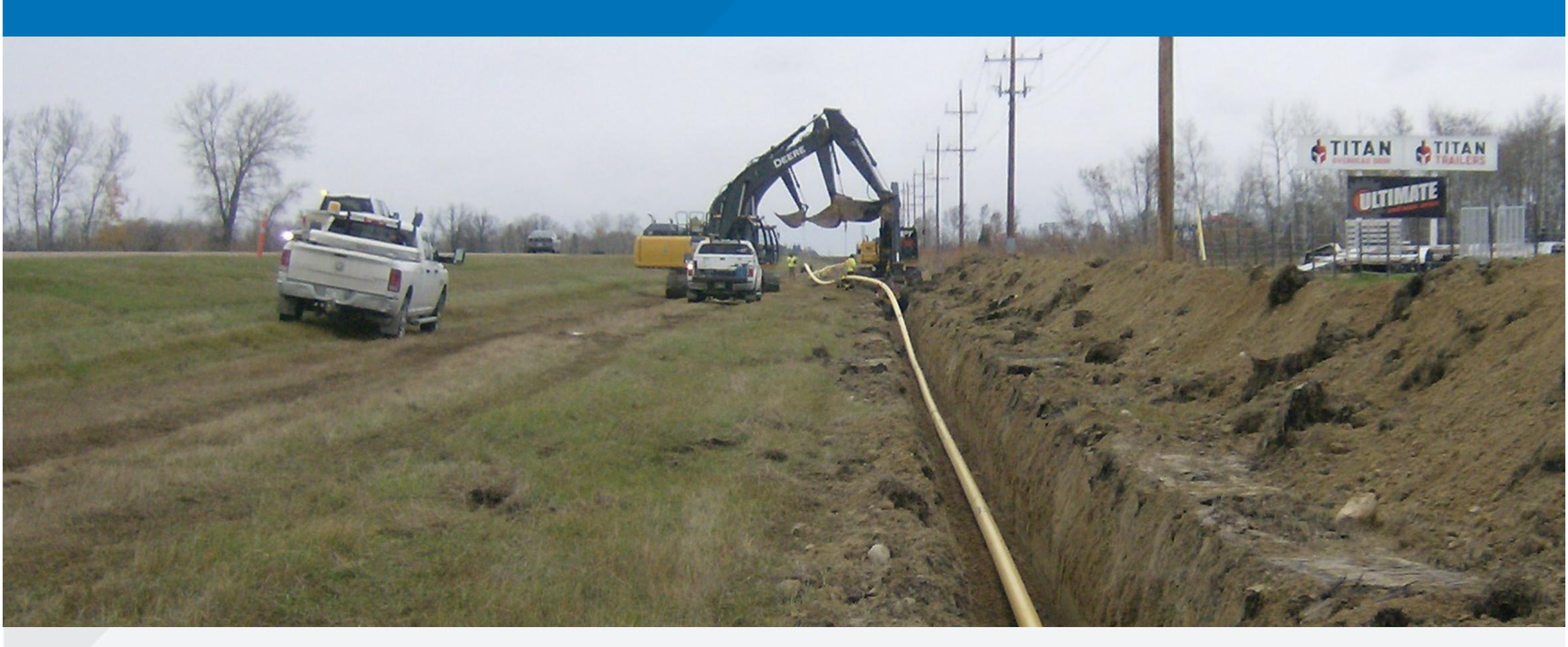
**Trenching** involves excavating the ground and placing the pipeline within the excavated area.
